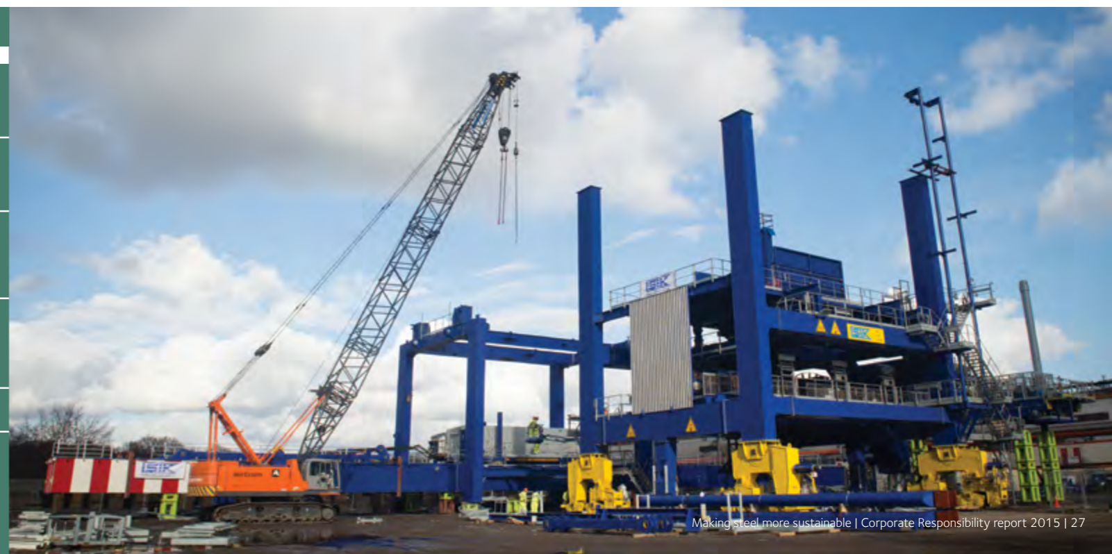
Assembly of a new harbour crane, equipped with a spray system to avoid dusting coming from raw materials.
