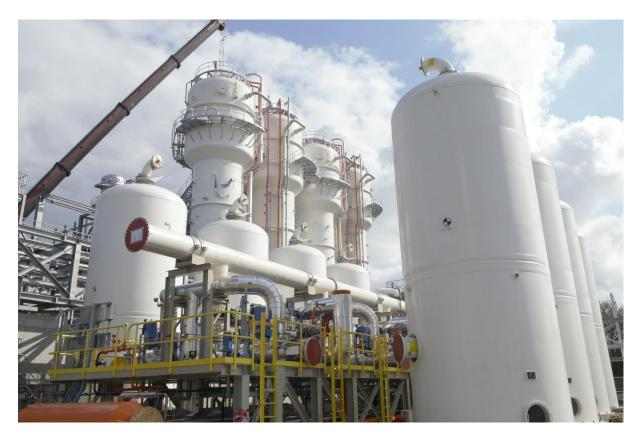
In April 2021, ArcelorMittal Belgium has marked a major milestone in the construction of its pioneering Steelanol project, with the arrival and lifting of four giant bioreactors at the Gent steel plant. The bioreactors, which will convert industrial gases captured during the steelmaking process into sustainable ethanol, are the central element of the installation.
